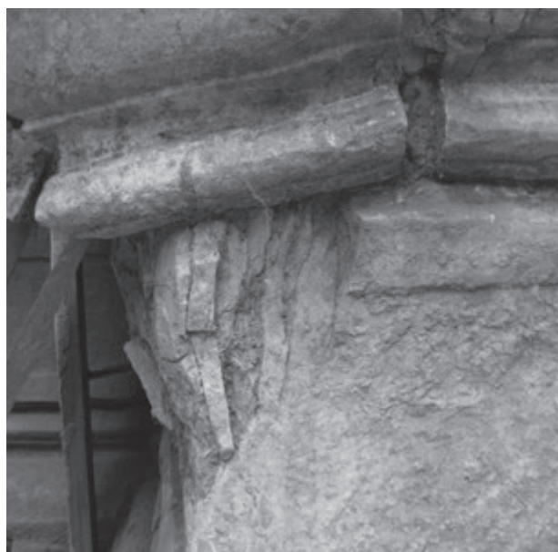
Fig. 39: Damage to a stone panel
