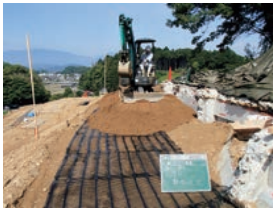
Fig.104 補強材施工状況
