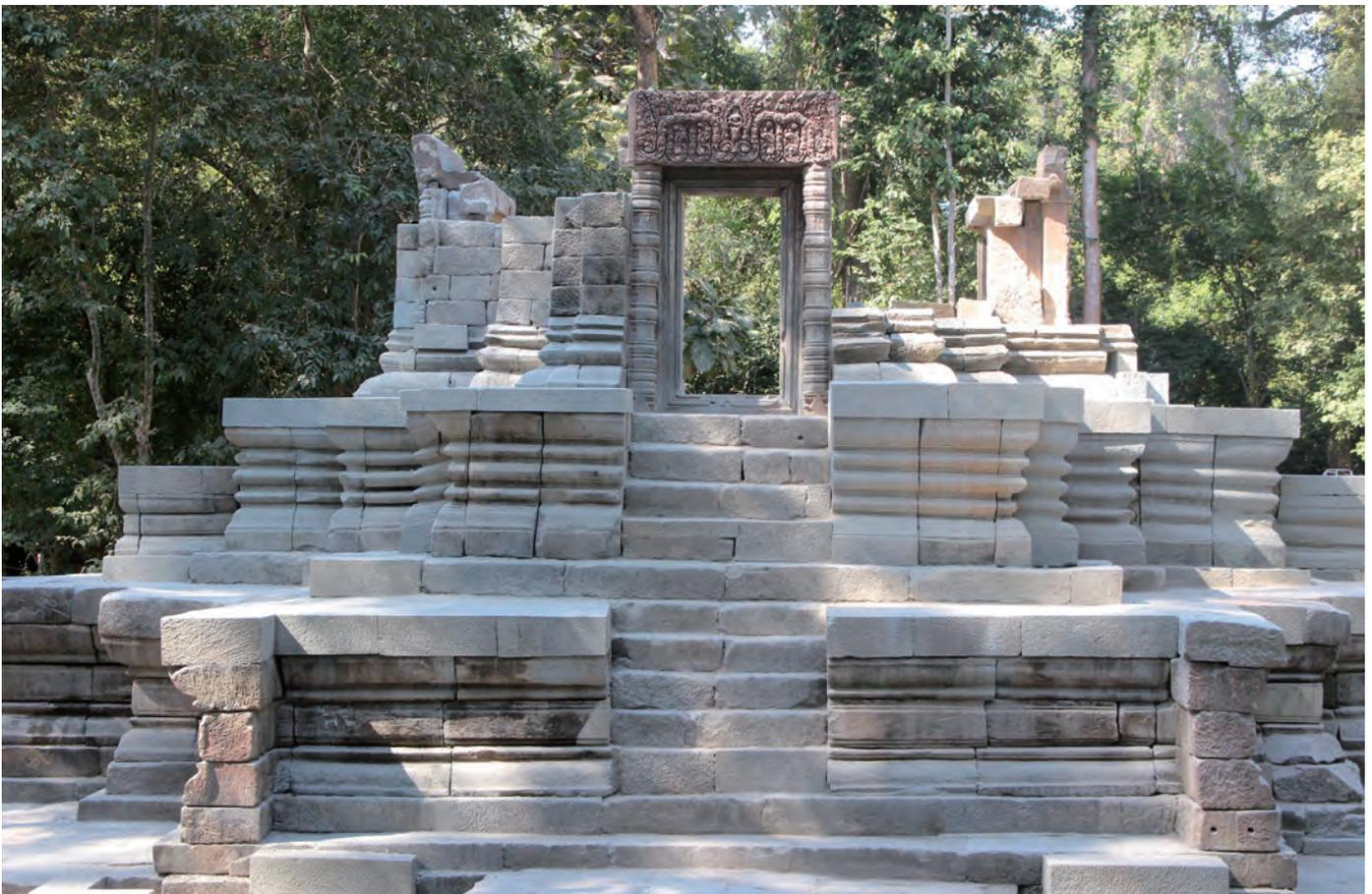
Fig. 29 View of the reassembled middle and upper platform and façade of the central sanctuary (view from the east)
