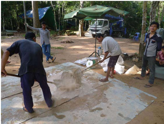
改良土を作るため、もともとの基壇盛土（粗砂）に若干の粘性土、消石灰およびラテライト粉末を混合する To consolidate the foundation soil, a small amount of clay, slaked lime and laterite powder were added to the original foundation soil (coarse sand)
