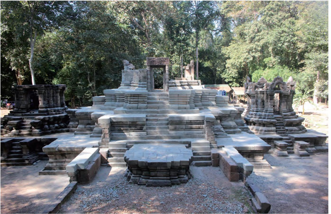
Fig. 28 View of the reassembled platform and façade of the central sanctuary (view from the east)
